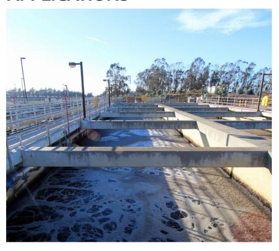
Wastewater applications require fast, precise control of air flow which in turn controls the dissolved oxygen (DO) in the aeration basin. Traditional control schemes result in DO measurements with large oscillations, requiring a higher DO setpoint. Large oscillations cause rapid wear of valves and other expensive system hardware while the supporting overranged DO setpoints create significant energy losses. Tighter control requires a faster, quieter measurement signal of the aeration air.
