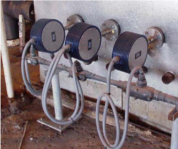
Figure A-5. Flex sensor connection for service loop, TA version using Liquid Tight Conduit.
