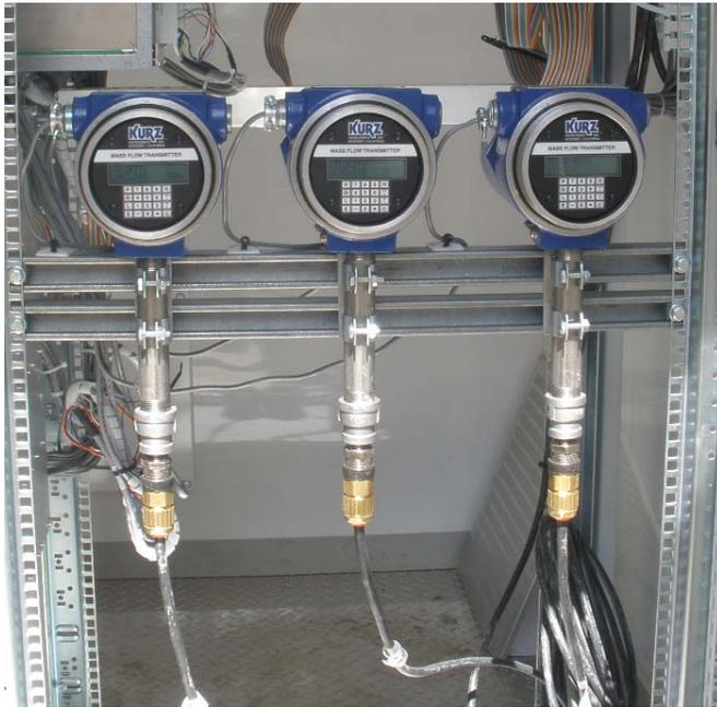
**Cable Gland Example with Braided Shielded cable on a TS configuration.**
