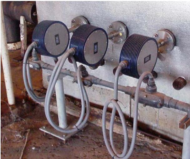
Figure AH-5. Flex sensor connection for service loop, TA version using Liquid Tight Conduit.
